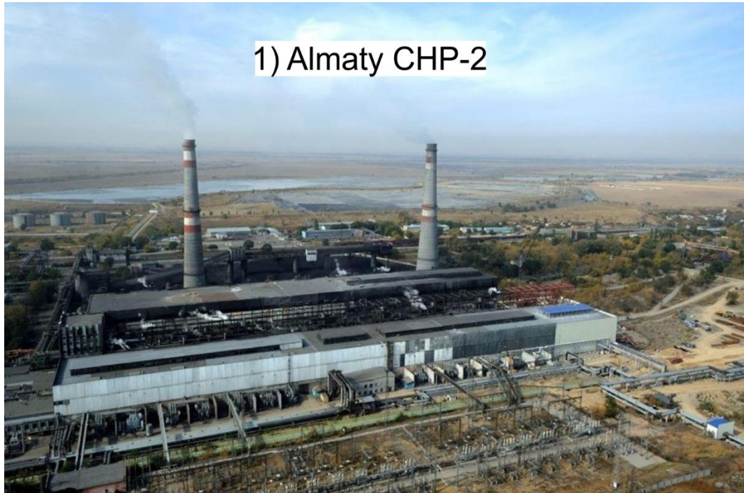
Figure 2-5: General look of the existing CHP-2 facilities and upon modernization
